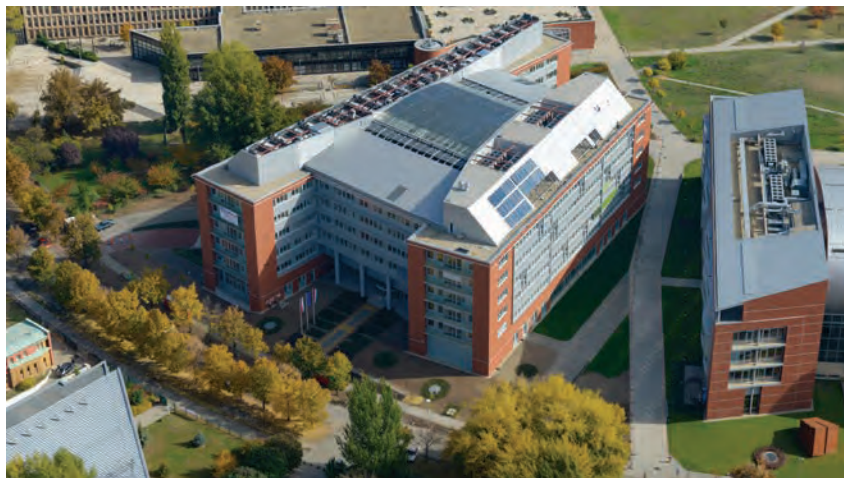
The new building of the Research Center for Natural Sciences of the Hungarian Academy of Sciences creates a strong potential for interdisciplinary research in molecular life sciences. The Center, with room for 400+ research personnel and state-of-the-art infrastructure, is located on the joint campus of major universities (Eötvös Loránd Science University and Budapest University of Technology).
